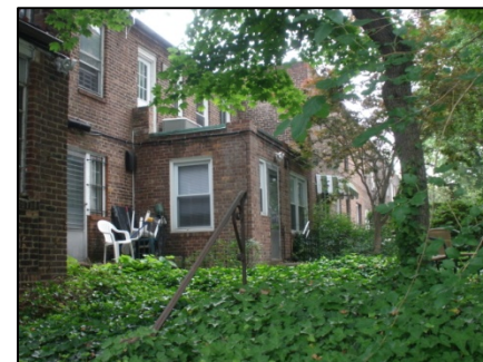
Rear yard additions or enclosed rear porches.
