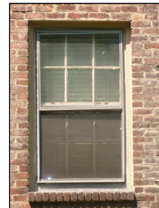
Figure 7: an original 6/6 double-hung window with a compliant storm window (LPC, 2007).
