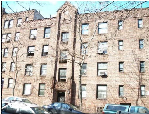
Figure 12: a decorative parapet that would require very careful restoration work (LPC, 2007).
